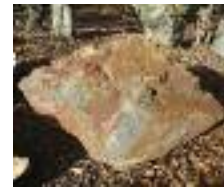
Slate with rust
